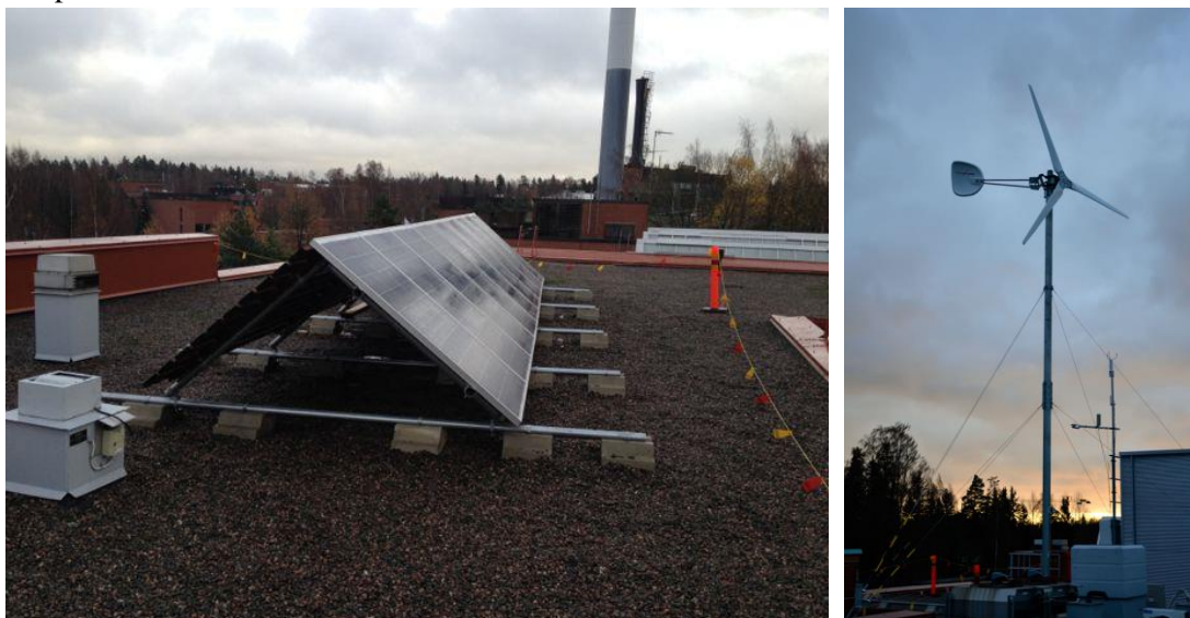
Figure 16. PV panels and microwind turbine on the roof of the K4 building.
