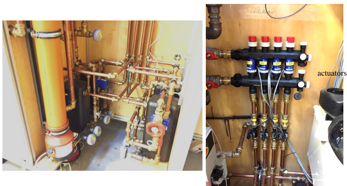
Figure 29. The heat exchangers emulating the heat emitters in a heating system (left). The actuators of the heating system (right).
