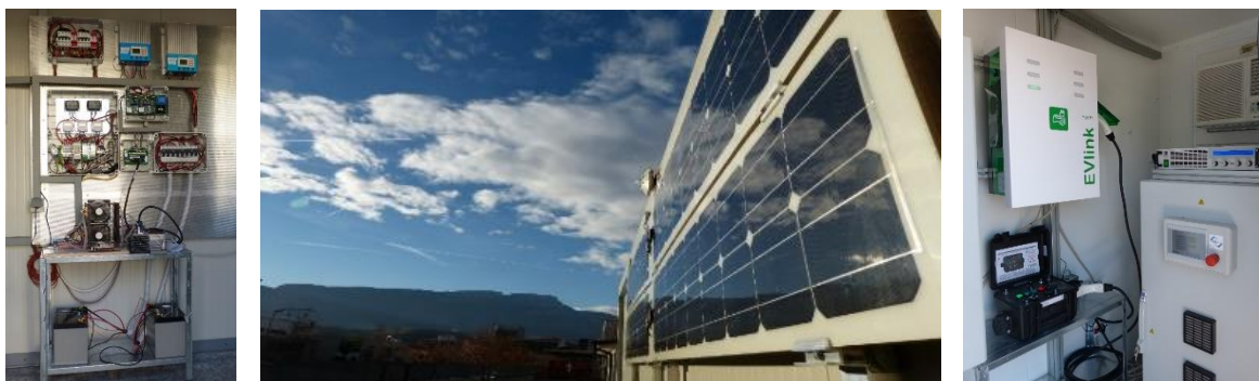
Figure 4. Running campaigns on PV+battery system (left) to match scaled down single user profile aimed at evaluating different control strategies and effect on component efficiency. Adding eV charging system and Innovative Energy Storage System (right) managed by iBEMS (EU FP7 CommonEnergy project, http://www.commonenergyproject.eu )
