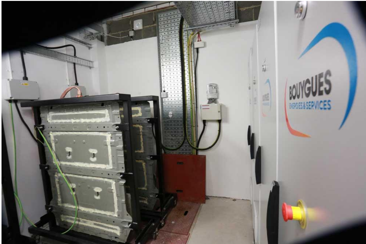
Figure 13.1 ELSA 2nd Life Battery Storage System.
