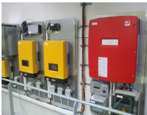
Figure 17. PV and island network inverters.
